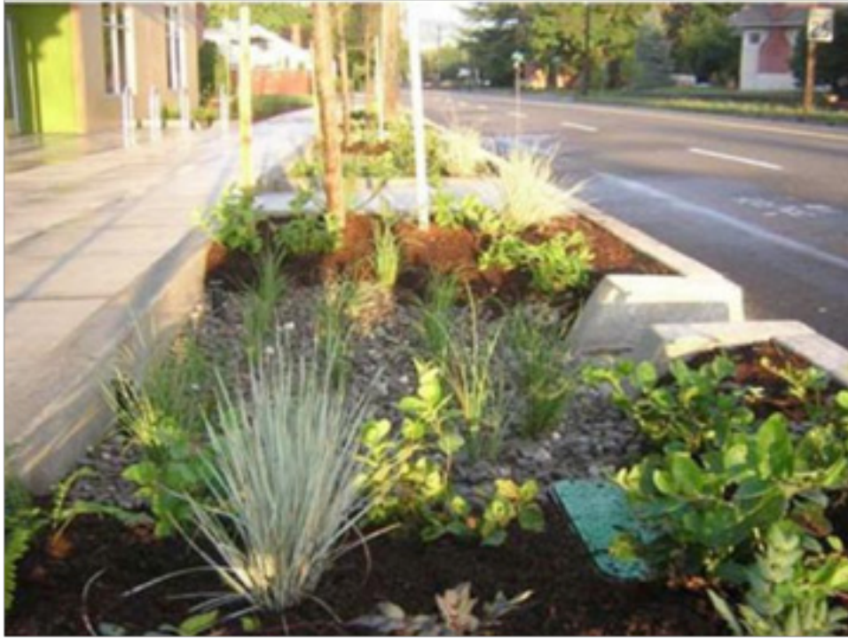
Figure 2: Bioretention swale: Portland, Oregon Courtesy: American Society of Landscape Architects HQs, Washington, DC
