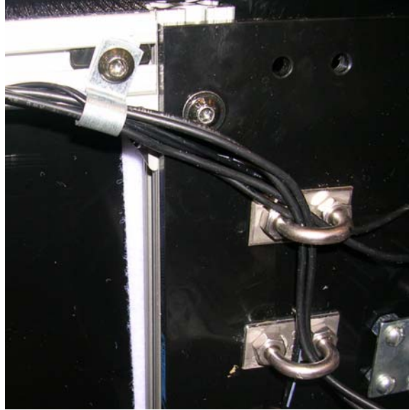
Figure 36: Organized routing of system wires
