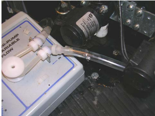
Figure 46: The left valve connection leak creates a small liquid pool on top plate
