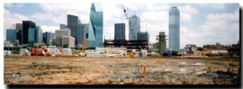
Jefferson North End during redevelopment
