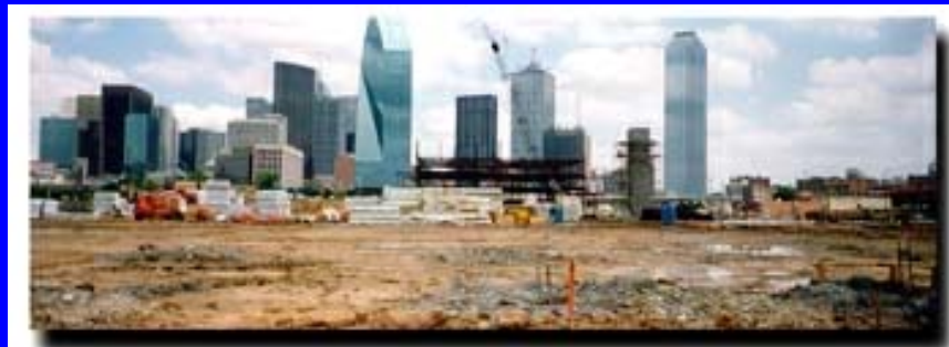
Jefferson North End during redevelopment
