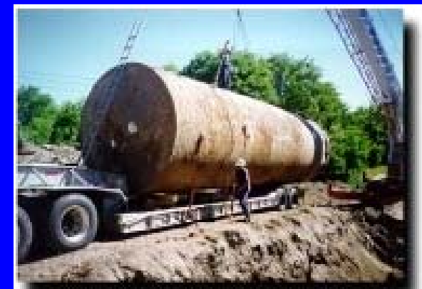
Underground storage tank removal
