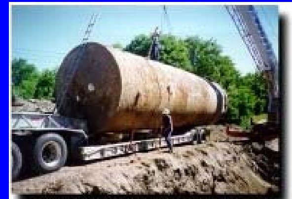
Underground storage tank removal
