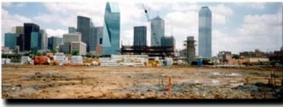
Jefferson North End during redevelopment
