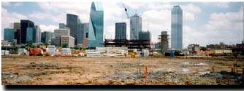
Jefferson North End during redevelopment
