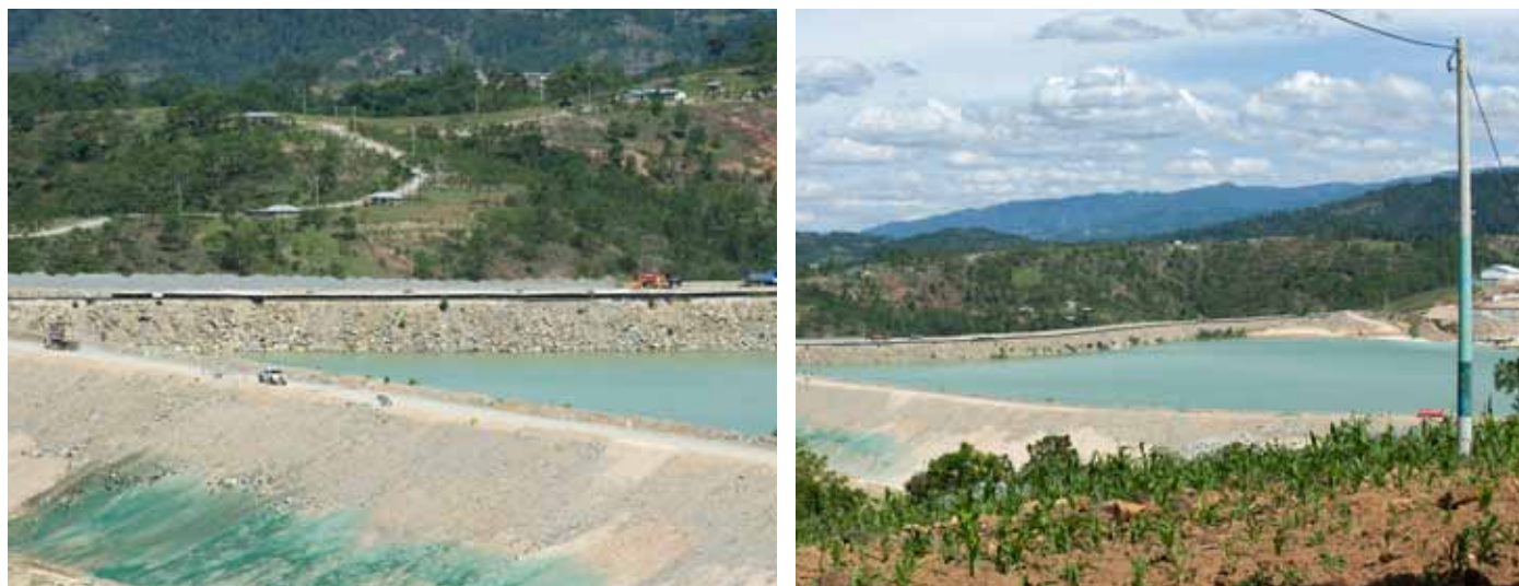
Figure IV.2 Marlin Mine: Tailings Pond
